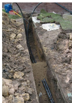
CORRECT GSHP TRENCH FOR LOOP & BACKFILL
