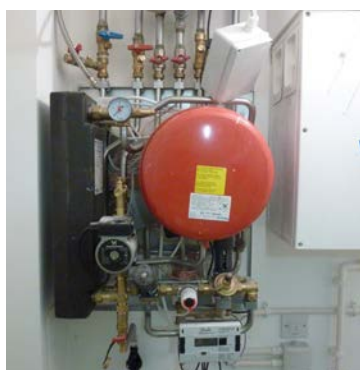
UN-INSULATED HEAT INTERFACE UNIT (HIU)
