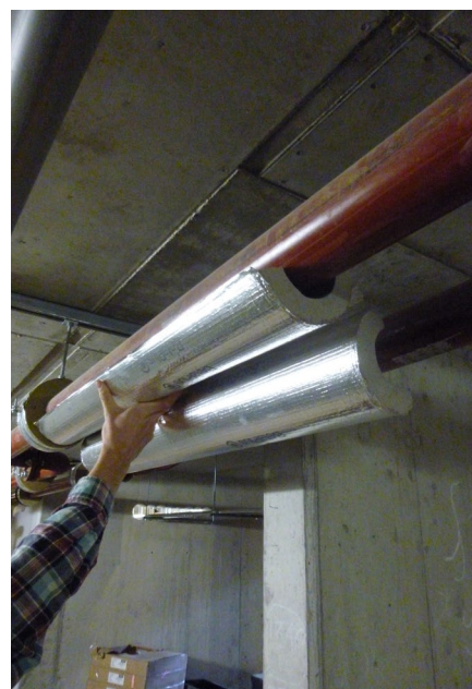
ADEQUATE INSULATION AROUND PIPES IN CORRIDORS AND FLATS
