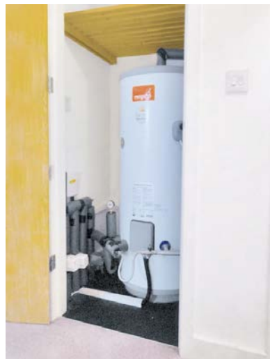
UNVENTED CYLINDER INSULATED AND LABELLED
