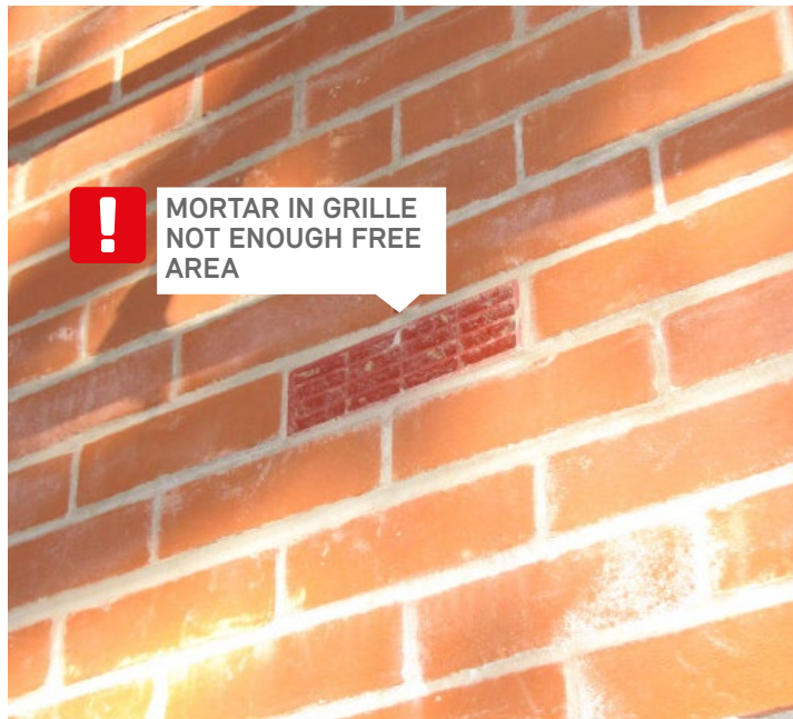
DUCT BEHIND AIRBRICK
