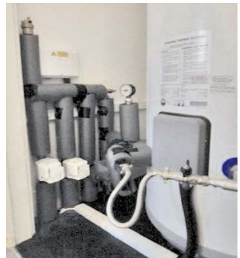
UNVENTED CYLINDER INSULATED AND LABELLED
