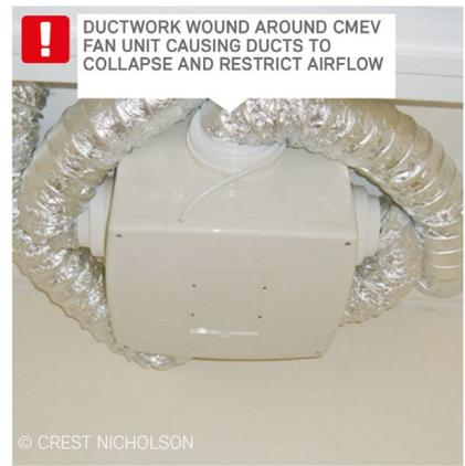
! DUCTWORK WOUND AROUND CMEV FAN UNIT CAUSING DUCTS TO COLLAPSE AND RESTRICT AIRFLOW
